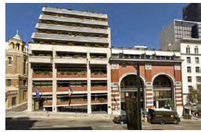
Picture 3 - The Building San Francisco Campus
