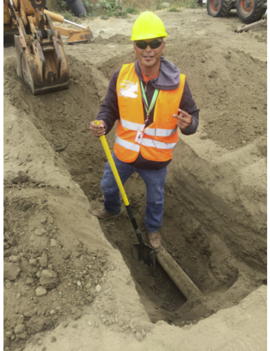
CIT student trenching, locating the pipe, and checking for appropriate shoring.
