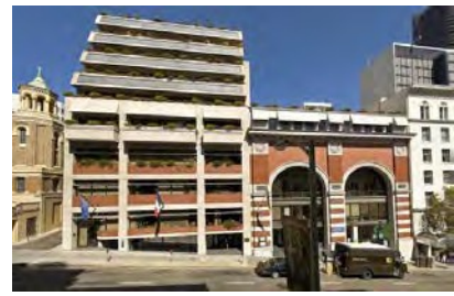
Picture 3 - The Building San Francisco Campus
