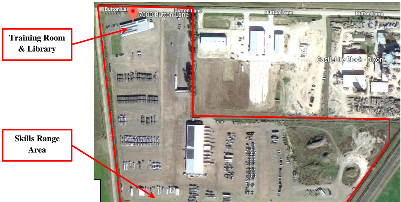
AAA Academy Facility within Button Transportation/Benjamin's Transfer Yard
