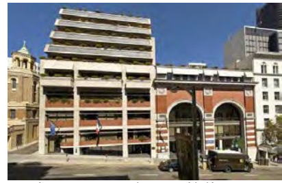
Picture 3 - The Building San Francisco Campus
