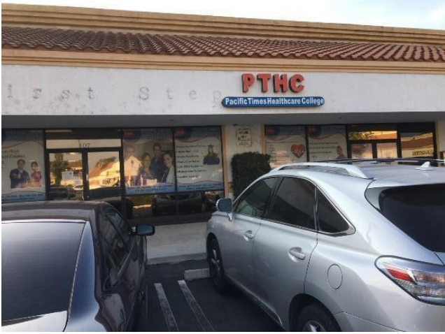
Front of Building
