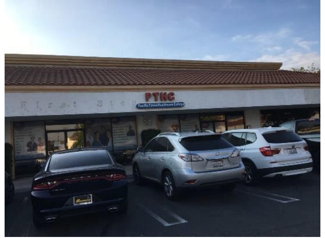
Front of Building
