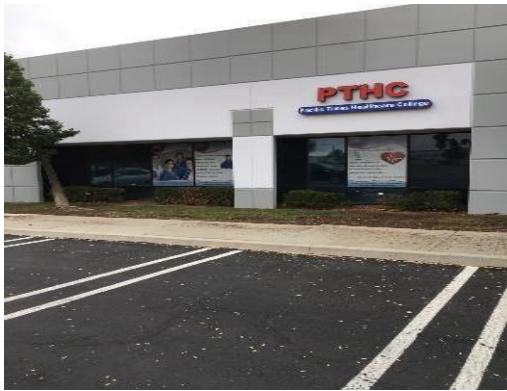
Front of Building
