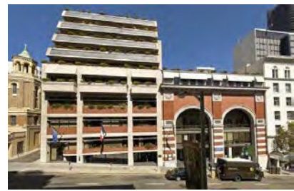
Picture 3 - The Building San Francisco Campus
